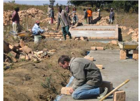
Jason+team laying foundations for the units.
