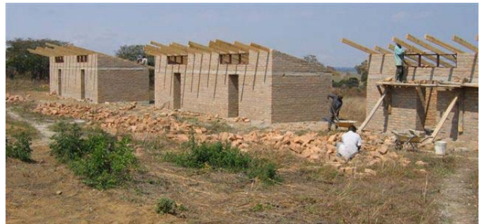
Dormitories ready for roofing at one unit.
