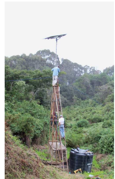
Mounting the Solar Panels was a tall order!
